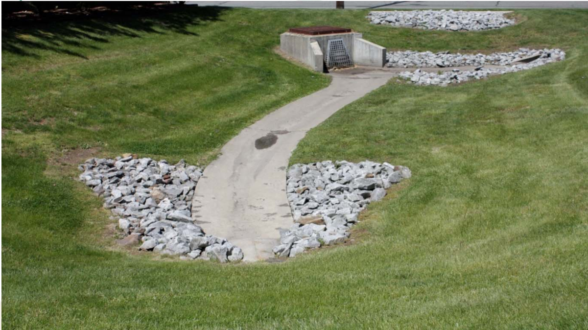
A well-maintained detention basin
