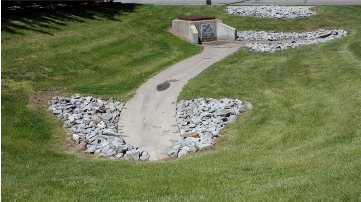
A well-maintained detention basin
