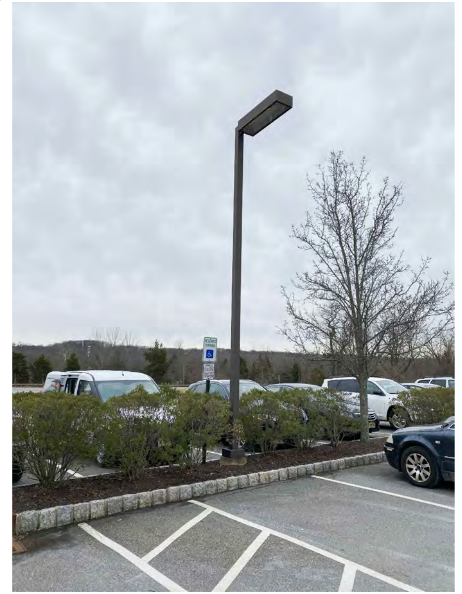
PHOTO OF A TYPICAL POLE-MOUNTED LIGHT FIXTURE WITH A SINGLE DOWNCAST FIXTURE. THE TOTAL HEIGHT OF THIS LIGHT IS 16' MAX. AND THE SIZE OF THE MOUNTING POLE IS 5" X 5".
