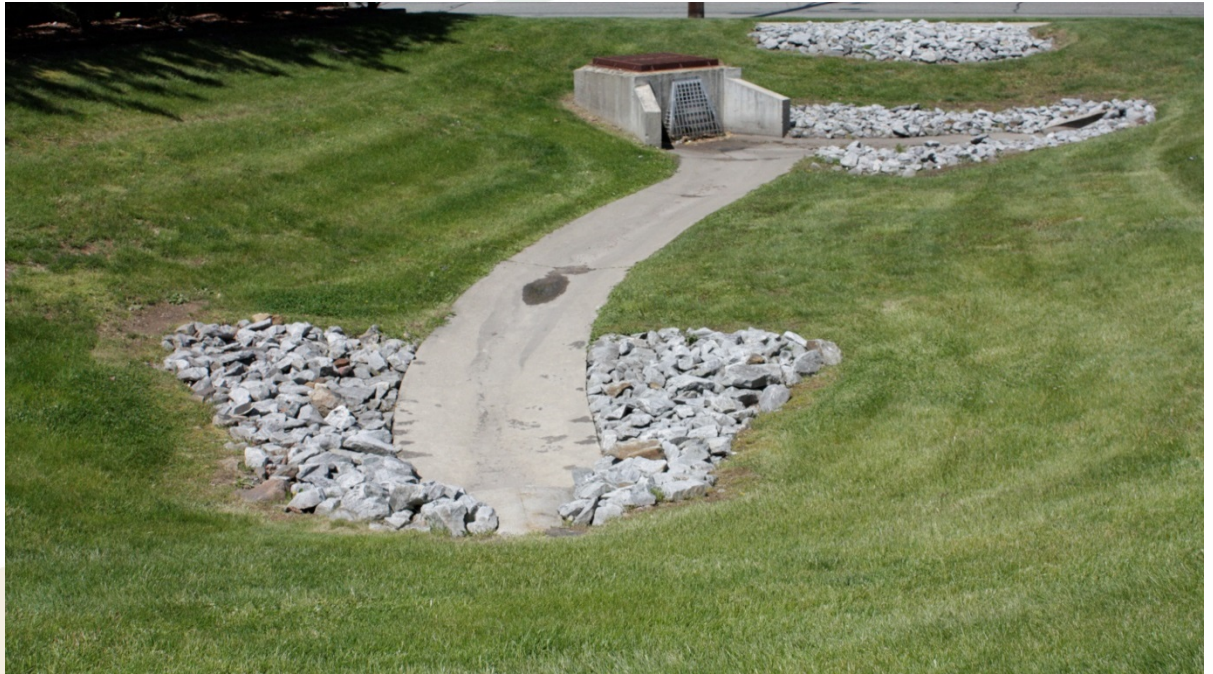
A well-maintained detention basin
